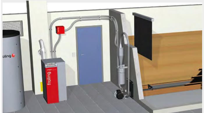
The Froling suction screw system is the ideal solution for rectangular rooms with front-end removal.
