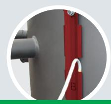
Correct positioning of the sensors on the terminal strip is crucial for optimal operation of the system!
