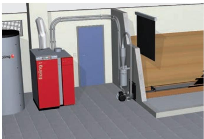
The Froling screw suction system is the ideal solution for rectangular rooms where front end removal is necessary. The deep and horizontal position of the discharge screw provides for the optimal use of the room space thus ensuring that a complete emptying of the storage is trouble free. In addition, Froling's suction system also enables a flexible boiler set-up.
